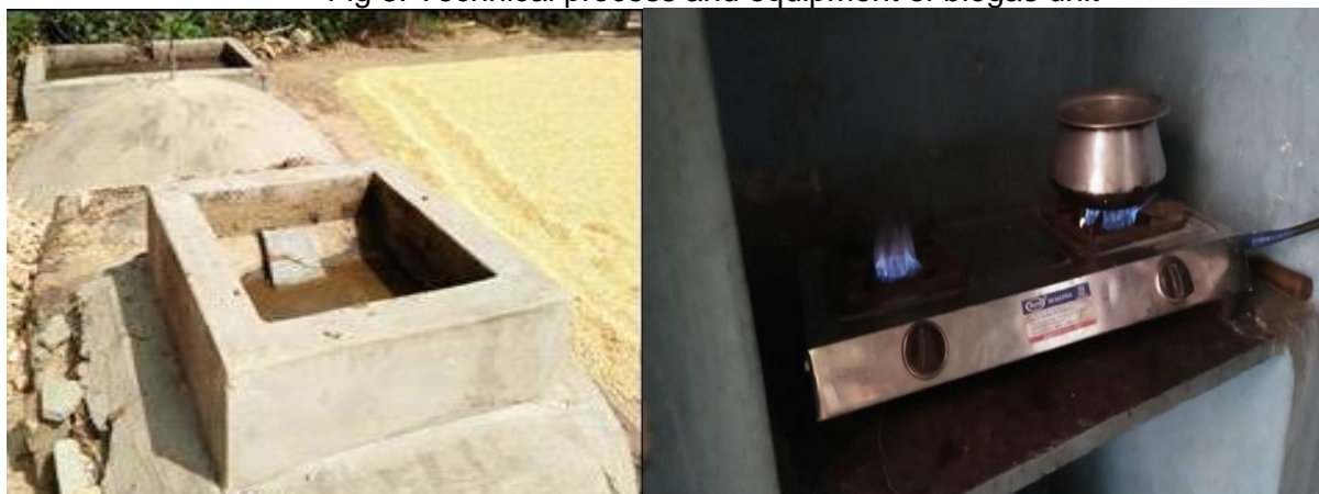
Fig 4: Constructed Deenabandhu Biogas Unit and Biogas Stove in the kitchen
